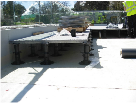
Second floor – precast pavers being installed on roof terrace
