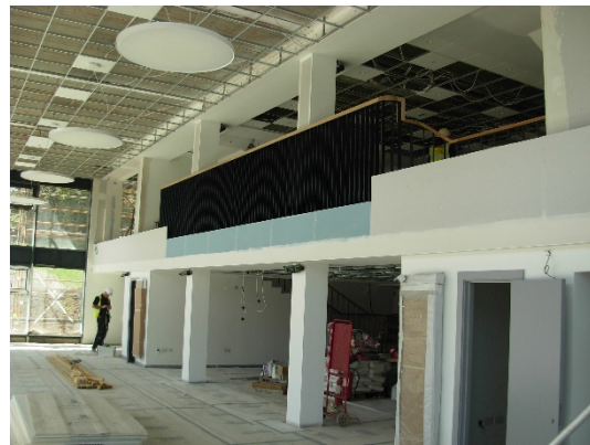
Ground floor café area looking up to first floor circulation
