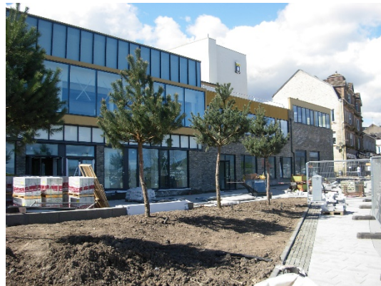
Eastern elevation – new glazed curtain walls, brickwork, cladding and public realm improvements (awaiting turf)
