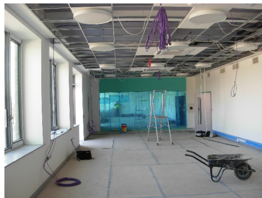
One of the two new fitness suites on the ground floor
