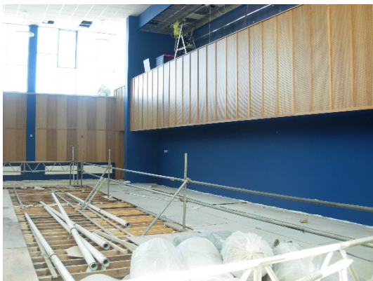
New Technical Gallery (top) with alcove underneath into which the retractable bleacher seating will fit. New solid oak to be installed and 'sprung floor' strengthened
