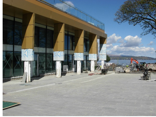
Southern elevation – new two storey glazed curtain wall and roof terrace, new clad columns (bottom two sections of cladding will be installed following completion of paving); new hard landscaping
